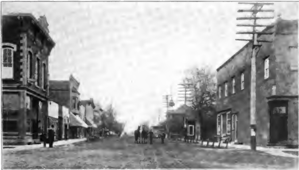
CLINTON STREET, LOWDEN
